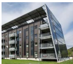
Retrofitted multi-family house Karfenberg (AT)
